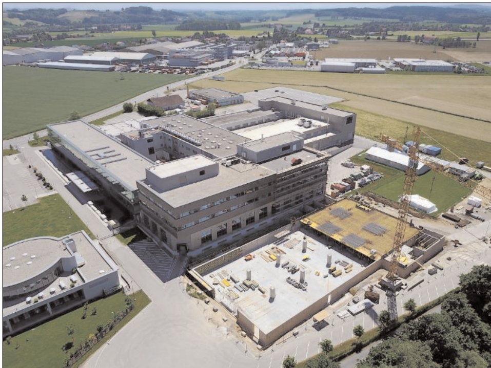
EVG's HQ, including construction site for additional production & test capacity.
