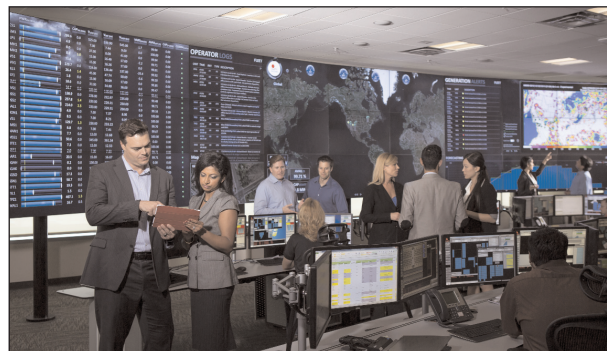
First Solar's NERC-registered Tempe-based US Operations Center.
