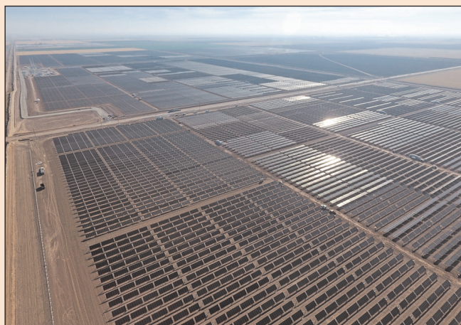
Solar Frontier Americas' completed Mustang Two solar project in Southern California.
