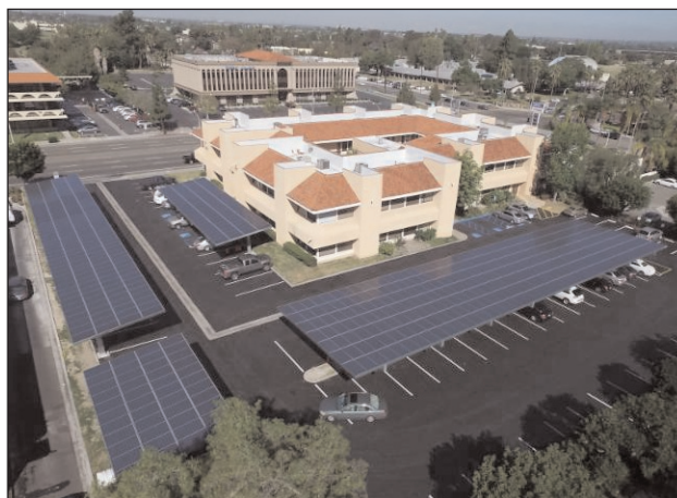
The 157kW Solar Carport Installation.
