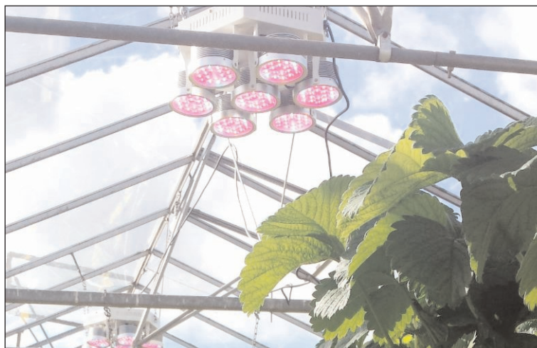
Plessey's PhytoLux Attis-7 LED horticultural lights, used by a commercial strawberry grower near Colchester, UK for season extension.
