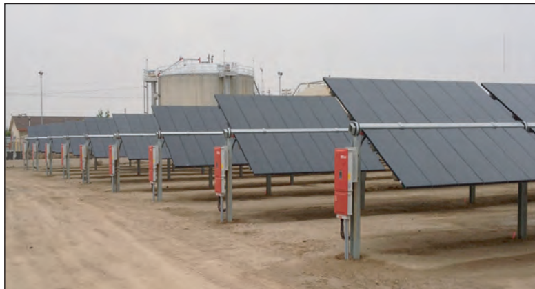
Stion's 255kW single-axis tracking solar project.
