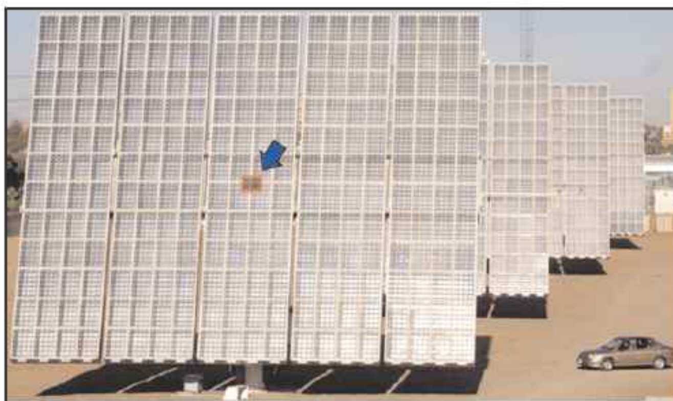
Amonix 7700 High Concentration Photovoltaic system. Also, by incorporating Amonix's patented
