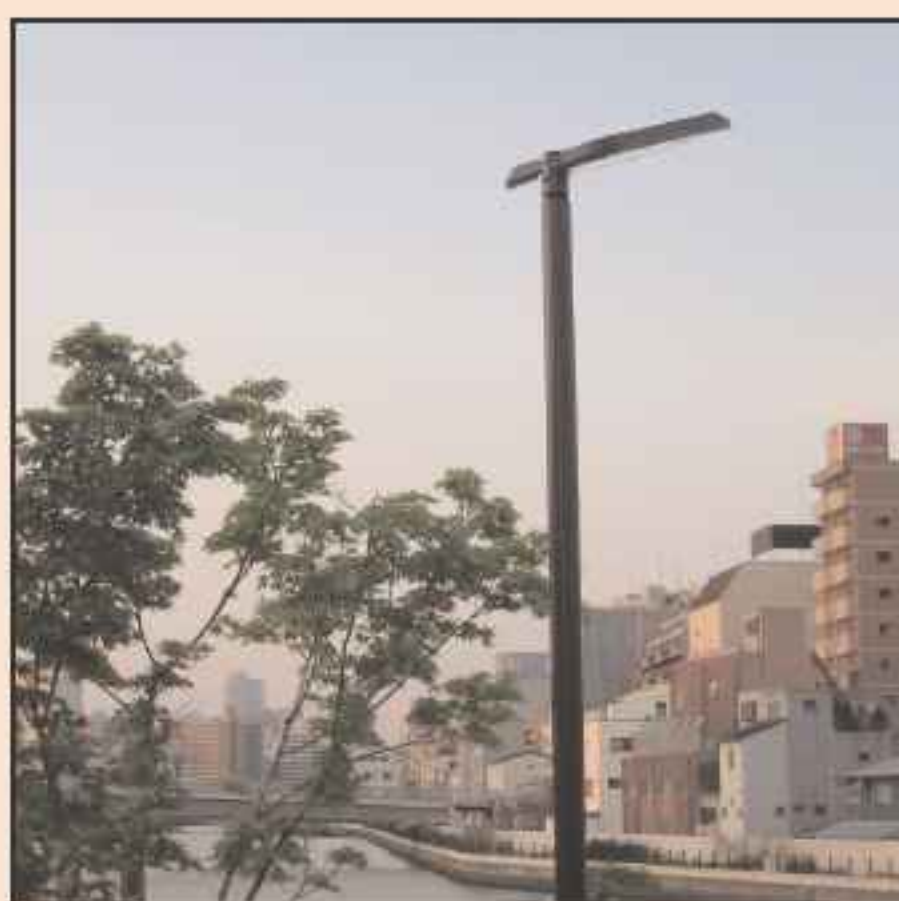
Street-lights in Osaka, Japan, each containing 36 cool-white Luxeon
