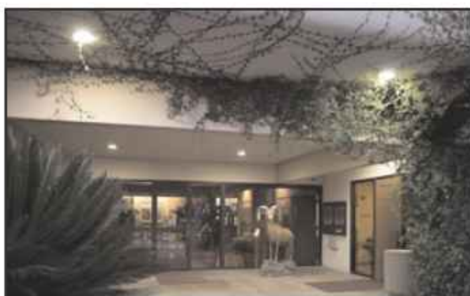
Exterior LED lighting at Indian Wells.
