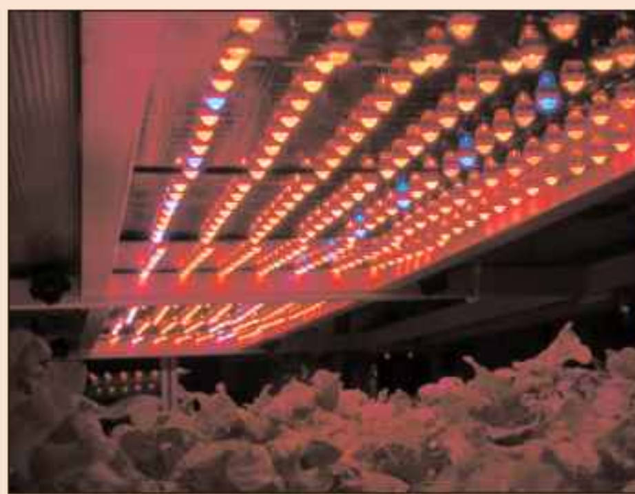
Red and blue LEDs used as an artificial light source for aiding the growth of plants.
