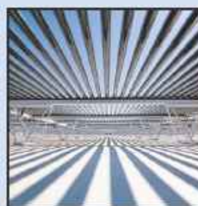
Cover: View from beneath an array of Solyndra's rooftop-mounted CIGS-based cylindrical solar modules, which can capture sunlight across a 360° surface capable of converting direct, diffuse and reflected sunlight into electricity, as well as allowing wind to pass through the array. p88
