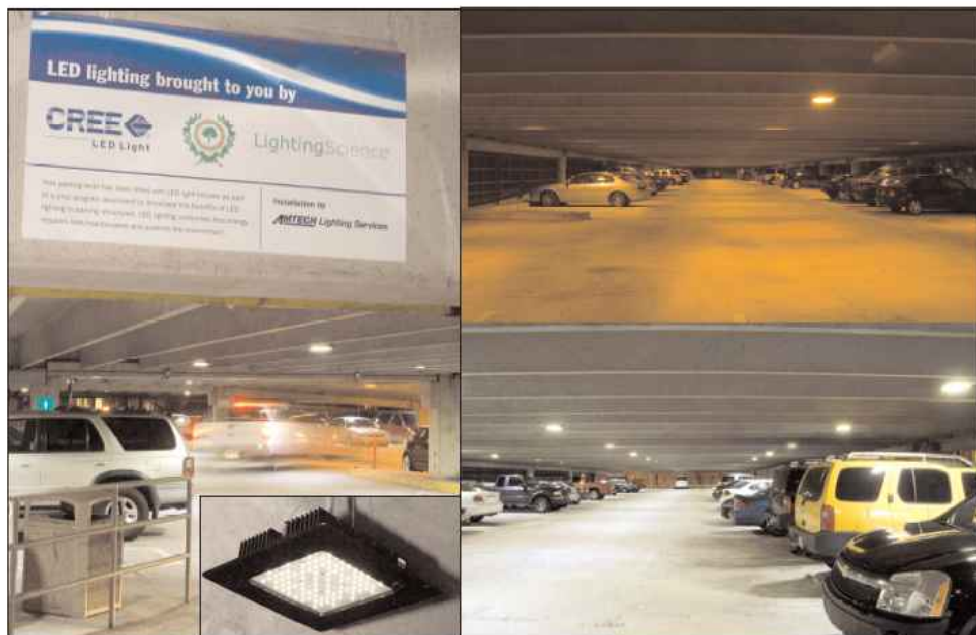
Garage before (top-right) and after (bottom) installation of LED lighting (inset).
