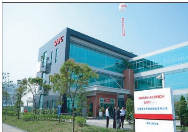
Exterior of the facility in Kaohsiung.
