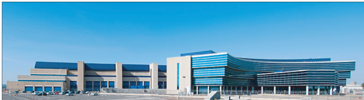
Profile of 3Sun's new integrated multi-junction, thin-film photovoltaic cell and module manufacturing plant.
