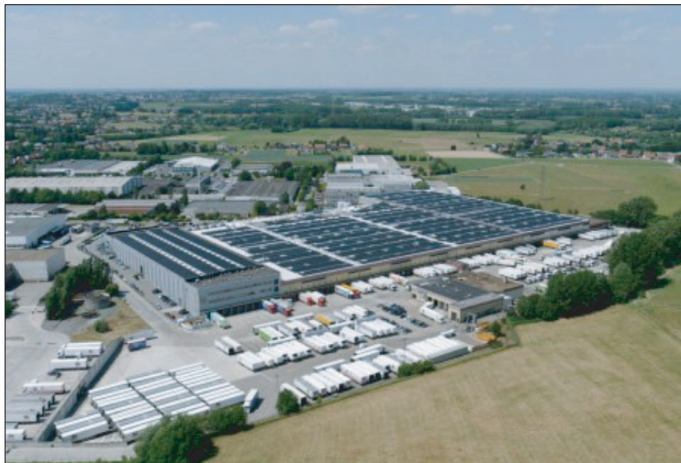
The 3MW Solyndra CIGS PV system on the distribution center roof in Belgium.
