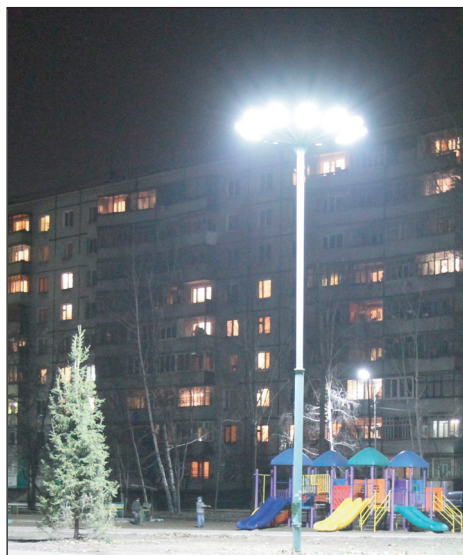
Street lighting using Osram Opto's Golden DRAGON Plus LEDs in Russian city Kazan.
