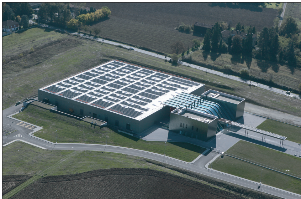
370kWp Solyndra system on a rooftop in the Piemonte Region of Italy.
