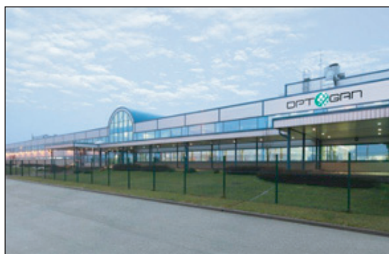
Optogan's new LED component and module factory in St Petersburg.
